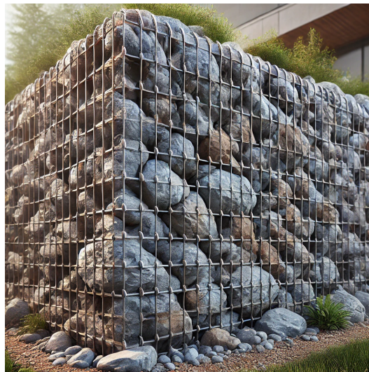
Figure 1. Our previous paper showed that gabion walls can provide effective ground vibration attenuation.
